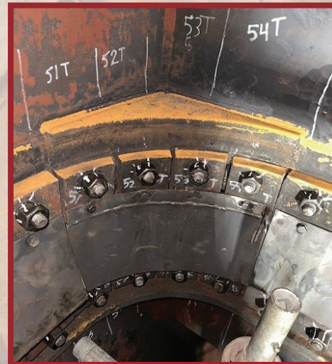
TURBINE CONDENSER DOG BONE EXPANSION JOINT
