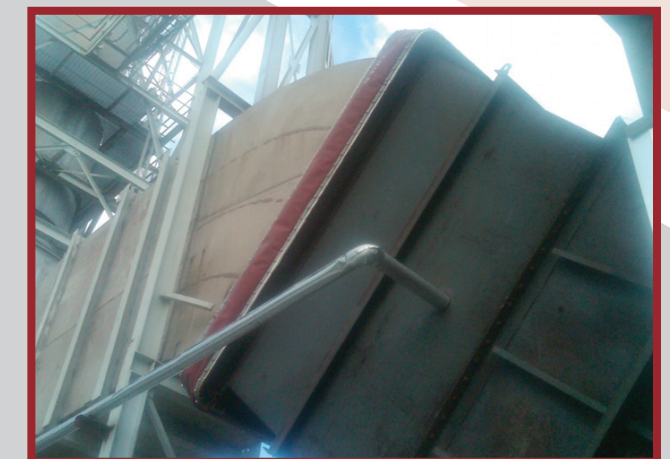
EXPANSION JOINT INSTALLED OVER METAL BELLOWS
