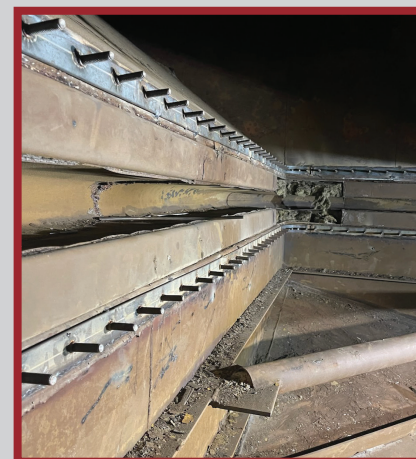
INTERNAL EXPANSION JOINT FRAMES AND FLOW LINER INSTALLS
