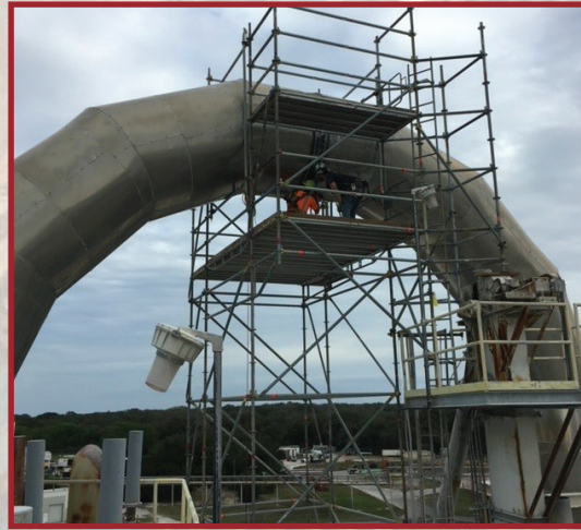
LIME KILN EXPANSION JOINT IN PROGRESS
