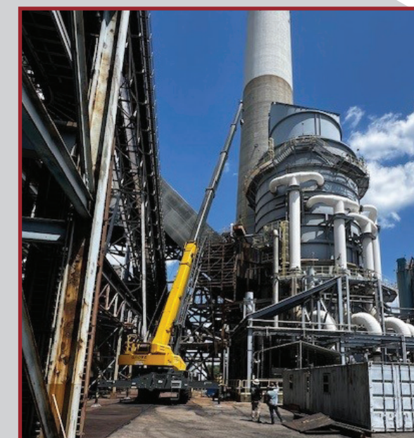
REPLACING SCRUBBER DUCT, EXPANSION JOINT FLANGE, EXPANSION JOINT AND FLOW LINER
