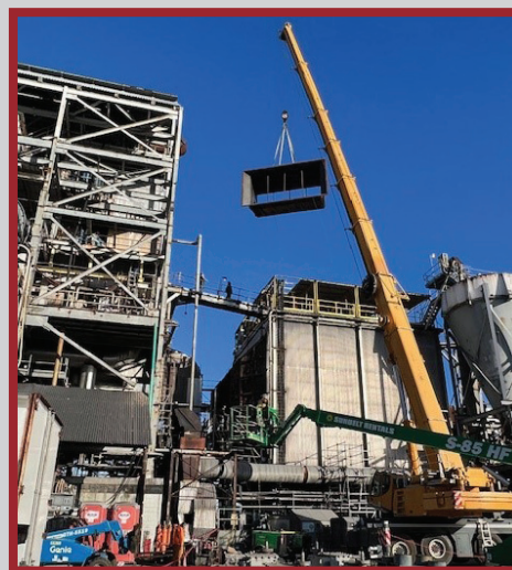
INSTALLING NEW PRECIPITATOR DUCT WORK WITH LARGE EXPANSION JOINT
