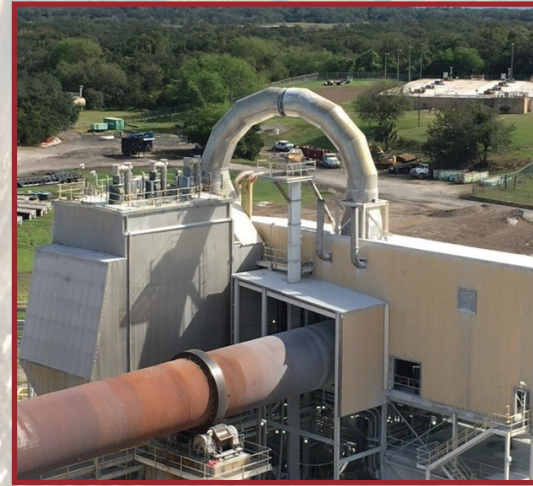
LIME KILN EXPANSION JOINT COMPLETED
