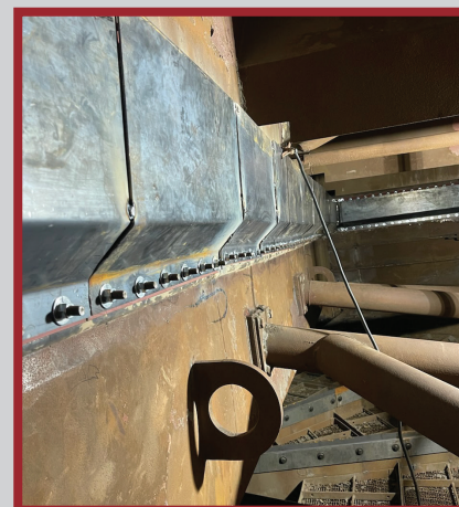
INTERNAL EXPANSION JOINT FRAMES AND FLOW LINER INSTALLS
