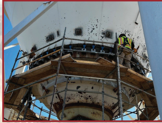
LIVE BOTTOM SILO EXPANSION JOINTS AND DOG BONE HANGERS
